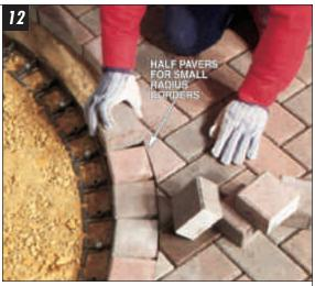
USE HALF PAVERS for bordering tight circles. Smaller pavers cut down on the size of the pie-shaped gaps between each piece.
