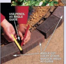
INSTALL THE BORDER, marking and cutting every other paver at an angle at curved areas.
