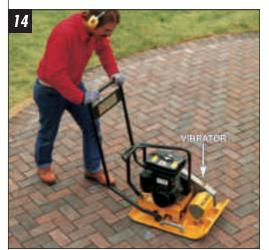
TAMP THE PATIO with a flat-plate vibrator after all the pavers are installed. Tamp entire outside edge first, then circle in.
