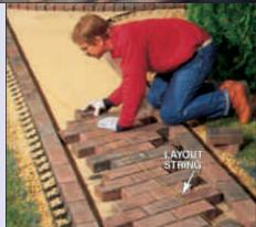
LAY THE PAVERS using a string for a guideline. Cut and install pieces that butt up to the border later.
