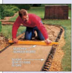
SMOOTH AND LEVEL the sand using a notched screed board riding along the edging for a guide. Include a slight tilt for good drainage.
