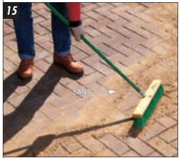
SWEEP COARSE, DRY SAND between cracks of pavers to lock them together and fill voids. Repeat with more dry sand in a few days.
