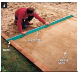
SPREAD AND LEVEL a 1-in. bed of sand over compacted subbase. Pipes provide a guide for dragging the 2x4 screed board across.
